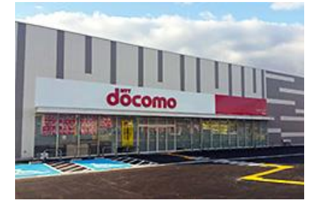
Iwade Store (Largest store in Wakayama Prefecture)
